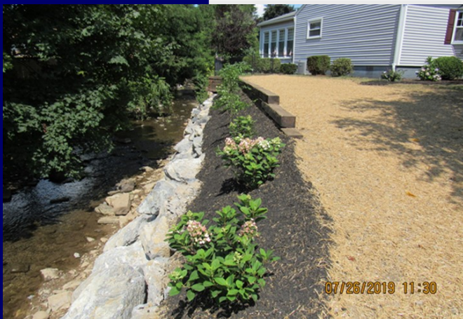
Spring Run after construction
