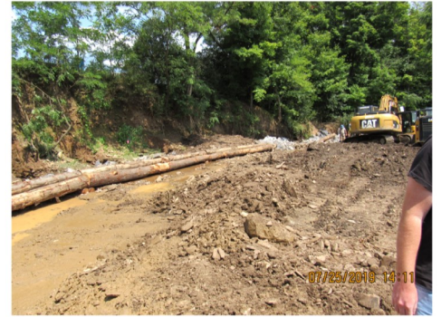
Installing mudsill
