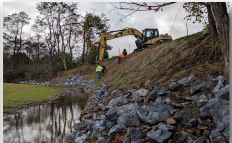
Spencer Run after construction
