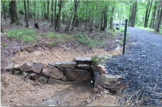
Stabilized Road and Culvert Endwall PA Game Commission, SGL 147
