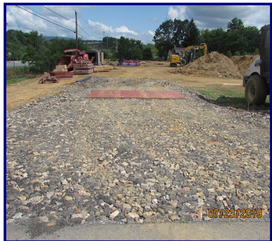
Rock Construction Entrances limit sediment from leaving sites during earthmoving
