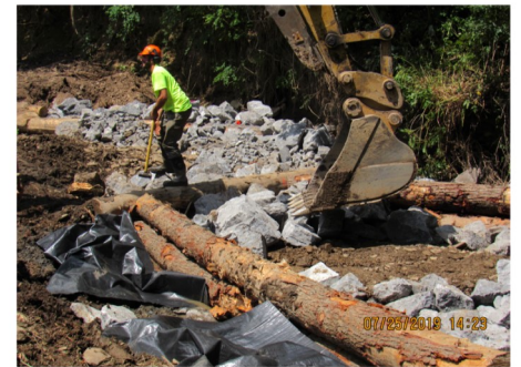
Installing Rock Vein
