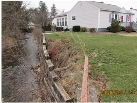
Spring Run site before construction
