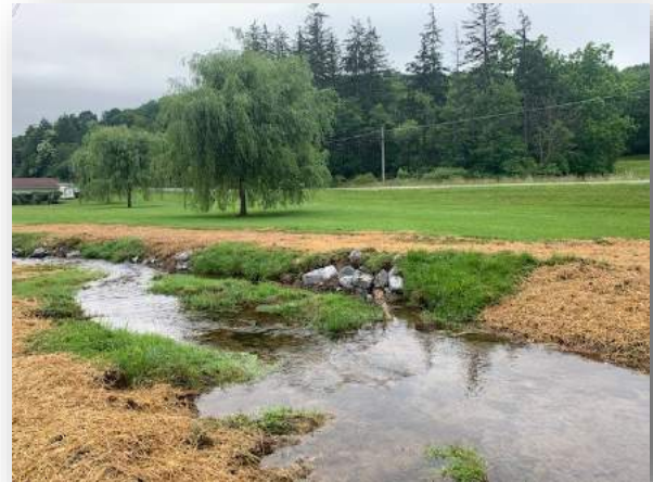
Maple Hollow Townhouse Property Gillans Run Streambank Stabilization Project
