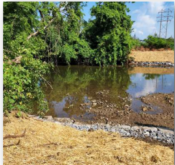
Streambank Stabilization and Stream Access at NatureWorksPark Beaverdam Branch of the Juniata River
