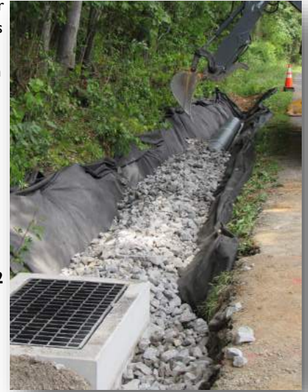
Drainage Project Miller Road Logan Township
