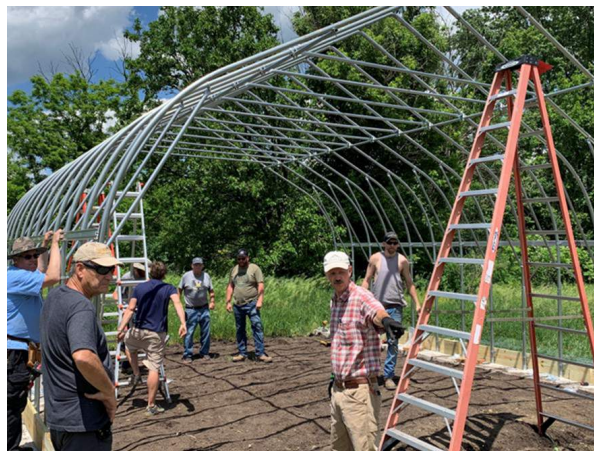
Hoop House Construction by Staff and Volunteers Summer 2022
