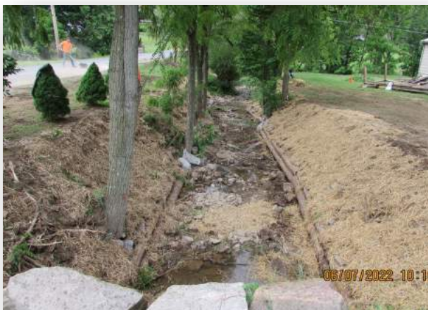
Yohn Property UNT to Spencer Run Streambank Stabilization Project
