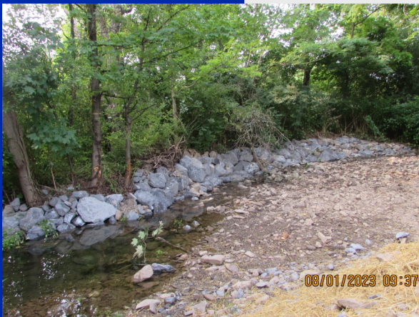
Stream Stabilization on Spencer Run
