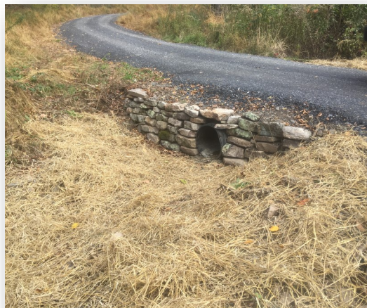
Stabilized Road and Culvert Endwall PA Game Commission, SGL 147
