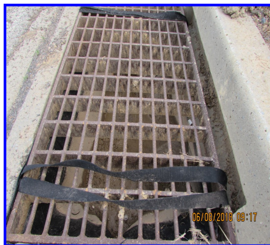
Inlet Filter Bag utilized to trap sediment until a construction site is stabilized
