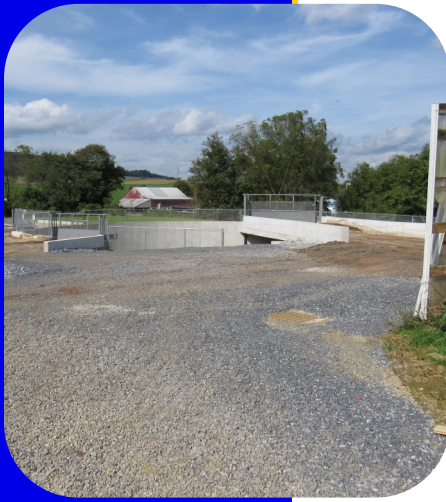
Manure Storage, Stabilized Access & Stormwater BMPs Planned and Implemented
