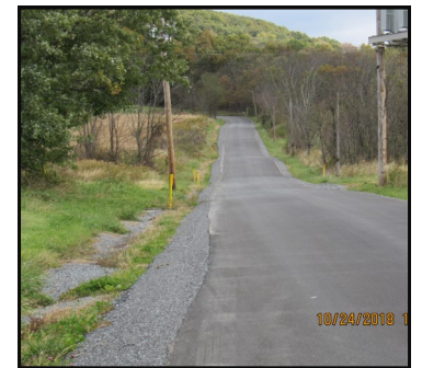
Completed Low Volume Road project Yingling Road– Taylor Township
