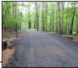
Completed Dirt and Gravel Road project Brubs Road– Pennsylvania Game
