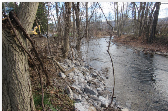
Poplar Run Streambank Stabilization Before and After
