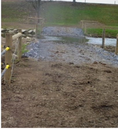
Stabilized Cattle Crossing and Fencing on Plum Creek
