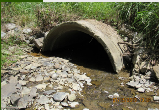
Undersized and Clogged Stream Crossing on Paw Paw Road Freedom Twp.
