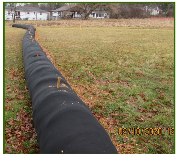
Compost Filter Sock installed prior to earth disturbance activity
