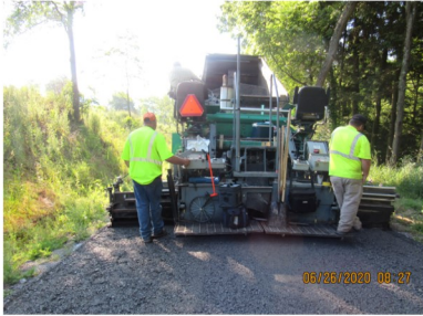
Paver Placement of Driving Surface Aggregate (DSA) Hemlock Lane Catharine Township
