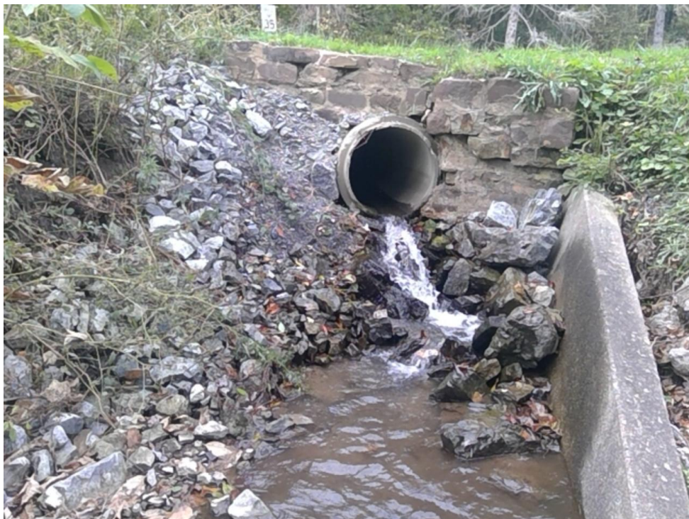
Photo 1: Crossing 1216 on Avalon Road is a severe AOP barrier.
