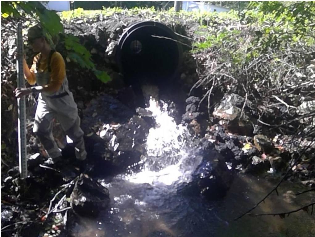
Photo 1: Crossing 1146 on Hollen Road. This crossing is a severe AOP barrier.
