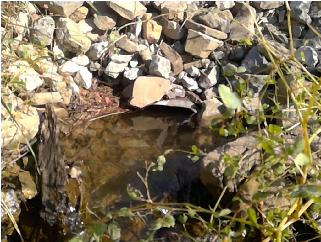
Photo 1: Crossing 1068 on Plum Creek Road. This crossing is almost completely filled with sediment and is a severe AOP barrier.
