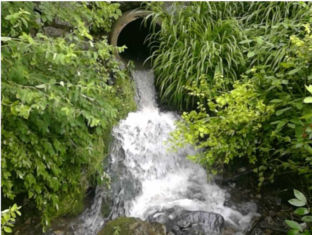
Photo 1: Crossing 905 on Bear Wallow Road. This crossing is severely constricted and is a severe AOP barrier.
