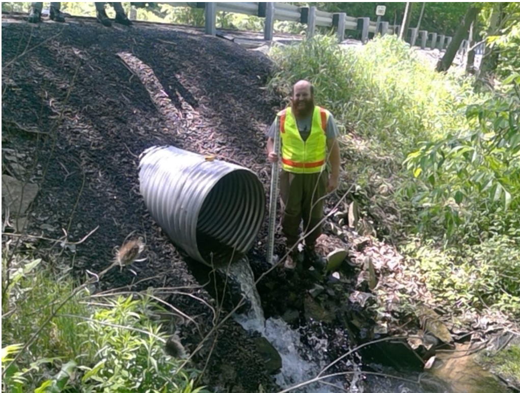
Photo 1: Crossing 691 on Knob Road has a perched outlet that causes a severe AOP barrier.
