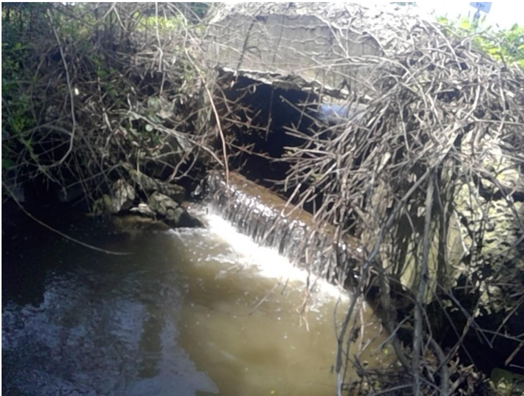
Photo 1: Crossing 851 on Shamrock Lane. The outlet of the box culvert causes it to be a severe AOP barrier.
