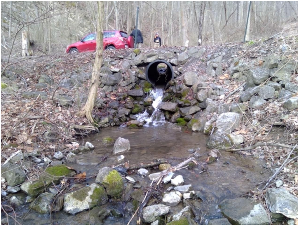
Photo 1: Crossing 635 on Wertz Road. This crossing is located on a UNT to Piney Creek. It is a severe AOP barrier.
