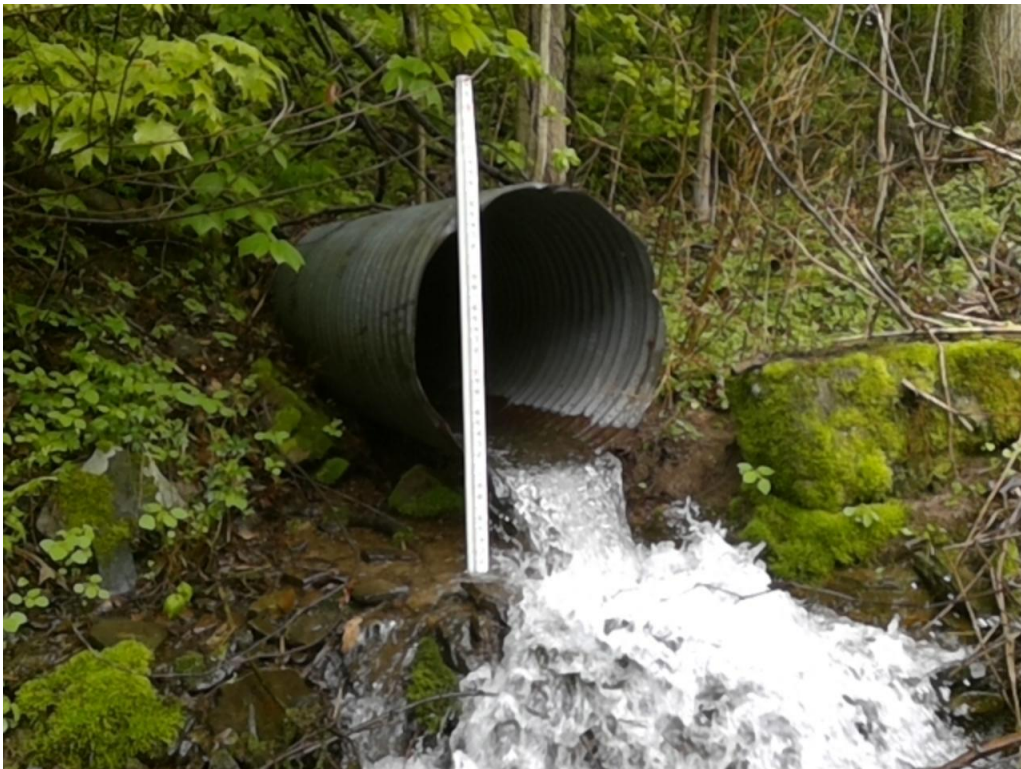
Photo 1: Crossing 644 located on Overland Pass. The culvert is severely constricted and is a severe AOP barrier.
