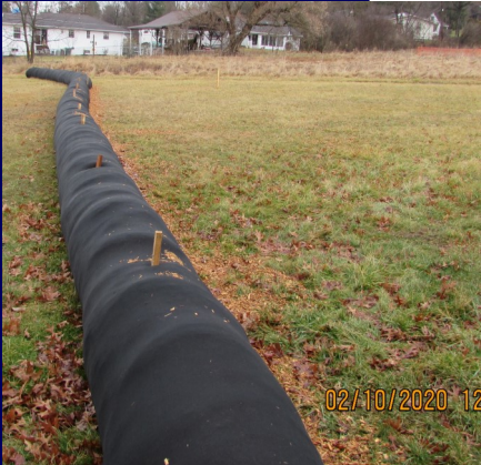
Compost Filter Sock installed prior to Earth Disturbance Activity
