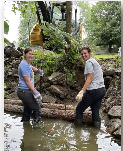
Tyne Blazier and Chelsey Weyant pinning logs for the Gillans Run Streambank Stabilization Project
